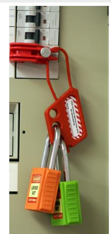
We recommend the use of LOK053 with the universal MCB lockout device.
