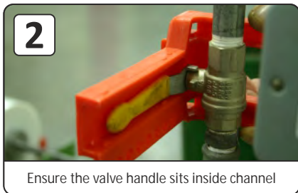
Place main body over the top of the valve handle, ensuring it sits inside the channel provided
